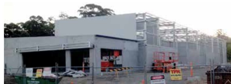
Above Left: The precast panels are installed and the Colorbond sheets are added as a feature.
