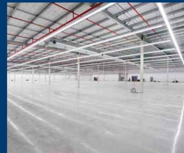
Left: Almost complete with final electrical work in progress in the main retail area.
