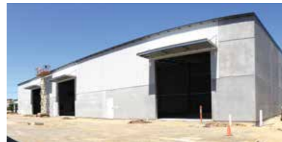
Above Left: The precast panels are installed and the Colorbond sheets are added as a feature.
